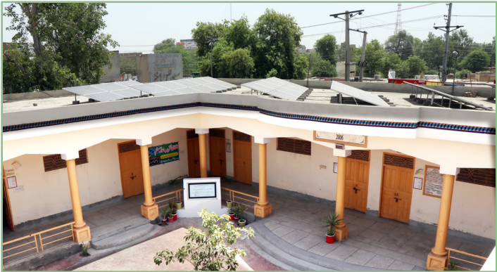
Installation of 31 KW Solar System Govt. MC Model High School, Burewala
