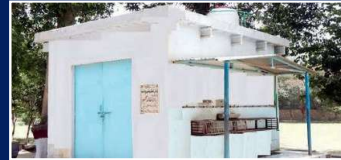
Water Filtration Plant Govt. Graduate College, Burewala
